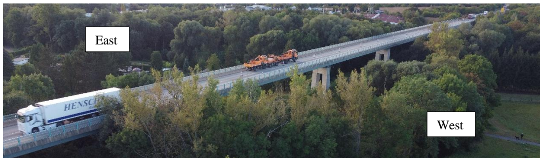
Figure 4: Picture of the Flossgraben Bridge. Trucks (additional mass) positioned at span 4.
