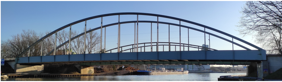
Figure 1. Sideview of the investigated steel arch bridge
