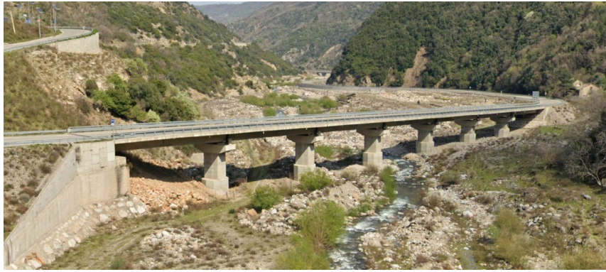
Figure 1: The Longobucco Bridge
