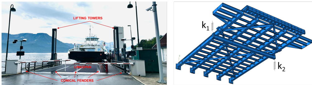
Figure 1. Magerholm linkspan and its finite element model (ABAQUS [7]).
