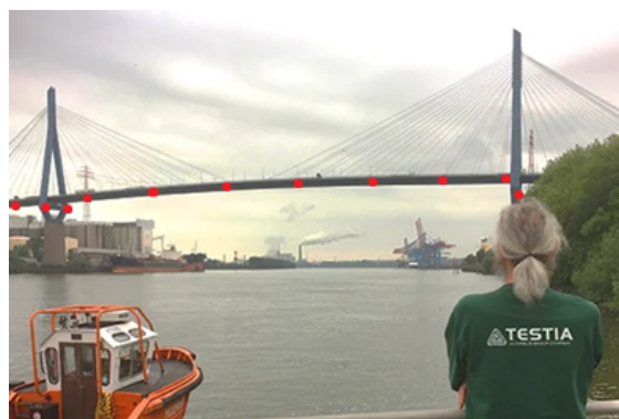
Figure 1. Global representation of a typical bridge work order where the red dots represent different sections of the bridge that are later up-scaled to extract exact sensor points [5]
