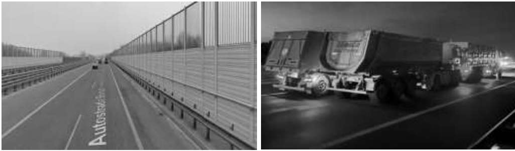
Figure 5. View of the structure under load.
